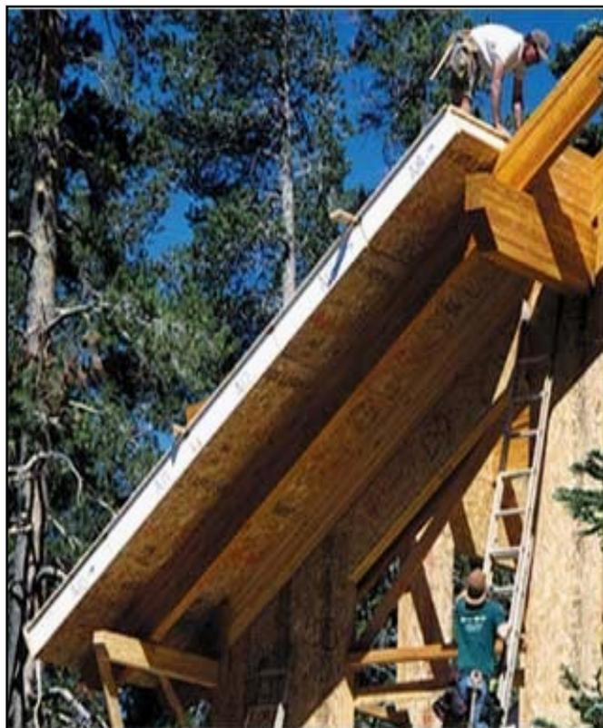
Structural Insulated Panels (SIPs) are composites of foam plastic [usually expanded polystyrene (EPS)] sandwiched between wood structural panels. Here, a SIP is used to build a roof.
